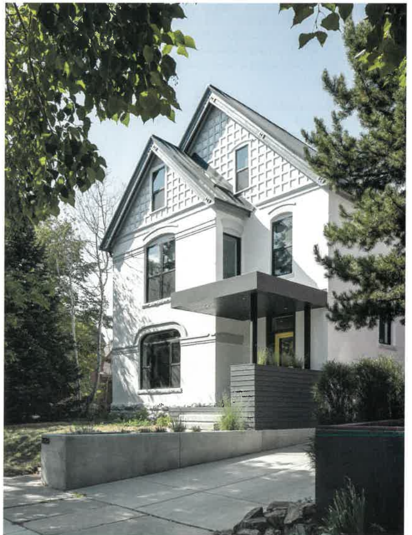
Right: The old Victorian home's new, metal-wrapped porch roof channels rainwater shed by the main roof down into concrete planters—watering the plants via perforated pipes—and out onto the street. A simple palette of light gray and white paints gives the structure a modern edge while highlighting the texture of its original details.
